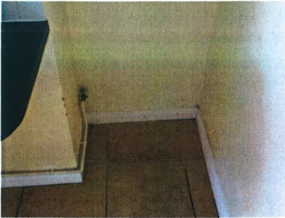
Photograph 7 – Kitchen (West Elevation side)
