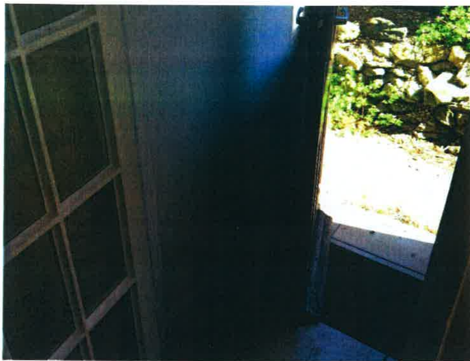
Photograph 9 – Rear internal hallway to South elevation
