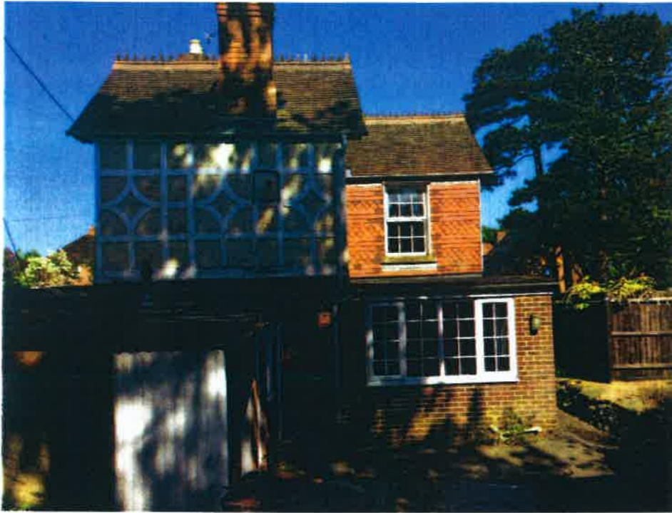
Photograph 3 – Rear (West) Elevation
