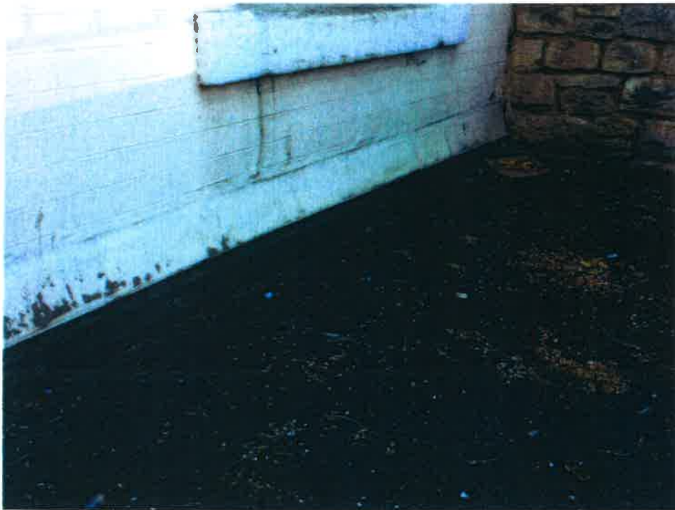
Photograph 20 – East Elevation - existing render skirt detail
