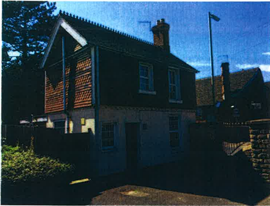
Photograph 1 – Front (East) Elevation
