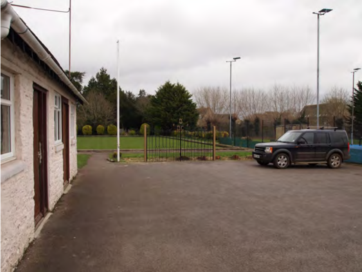
Image 1 – View from carpark and remaining metal gates
